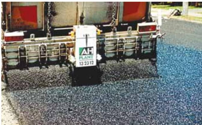
**Figure 9.** Example of a two-coat seal (VicRoads<sup>15</sup>).
