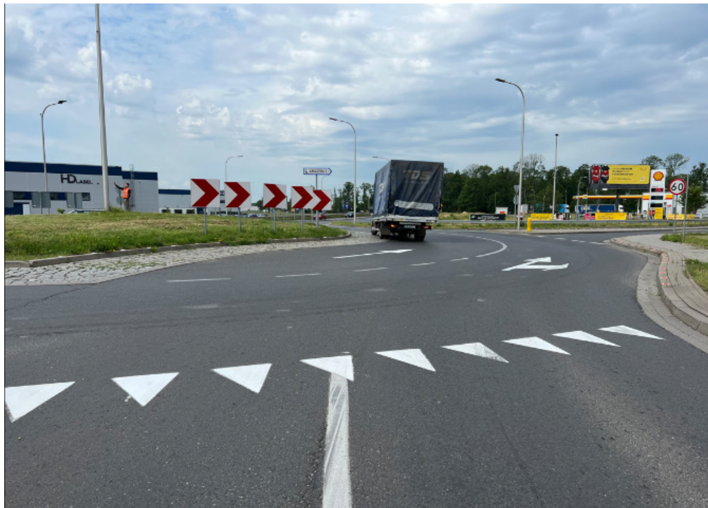
Figure 14: A series of large chevrons in the center island at a roundabout in Poland (Source: FHWA)
