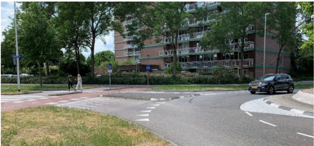
Figure 21: Raised pedestrian and bicycle crossing in the Netherlands (Source: FHWA)
