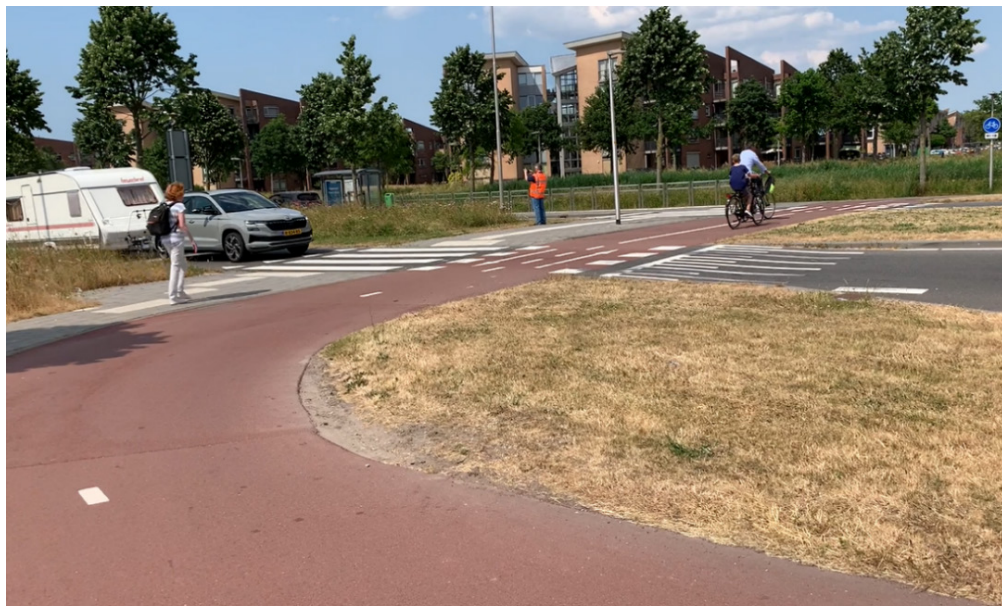
Figure 19: Typical separated pedestrian and bicycle facilities on the approaches to roundabouts in the Netherlands (Source: FHWA)
