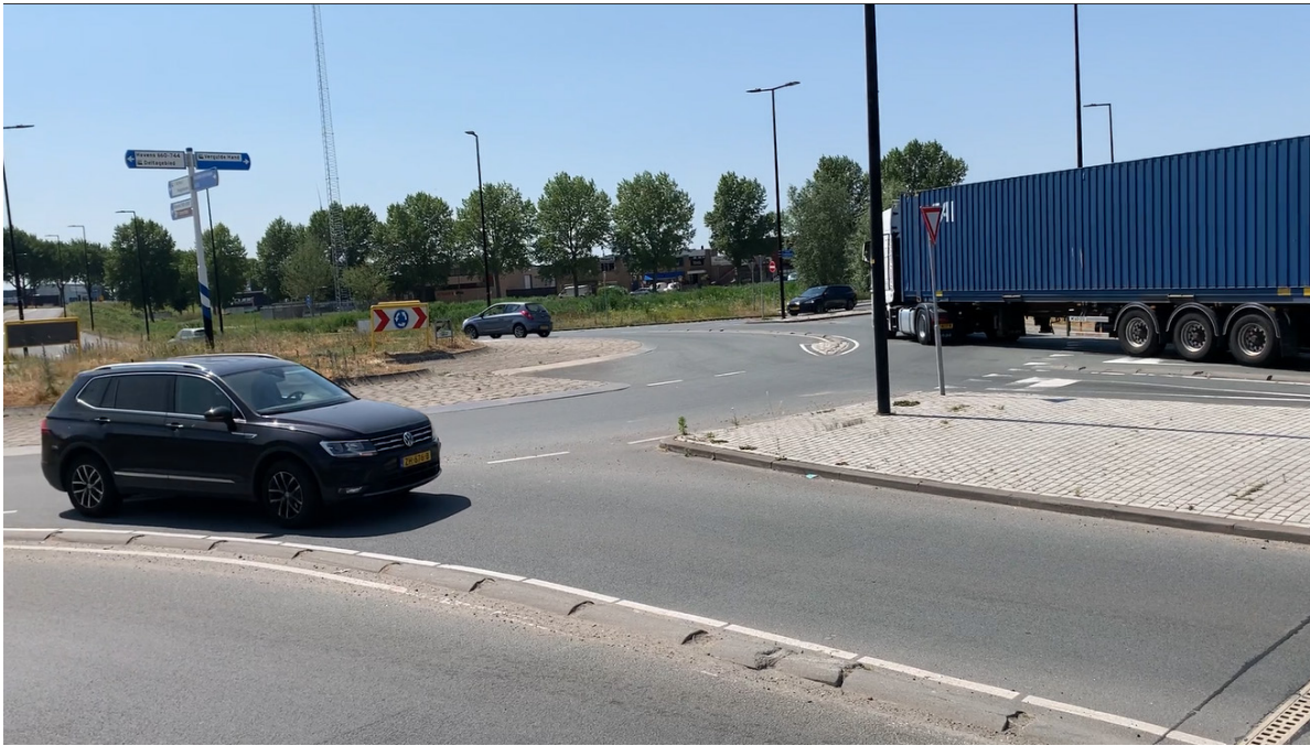
Figure 9: Raised channelization on the exit (forefront), entrance (near truck), and circulatory roadway with a right-angle inner lane in the center island in the Netherlands (Source: FHWA)
