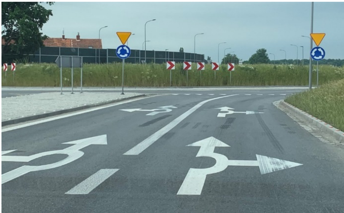
Figure 16: Example of entry signing and markings at a turbo roundabout in Poland (Source: FHWA)
