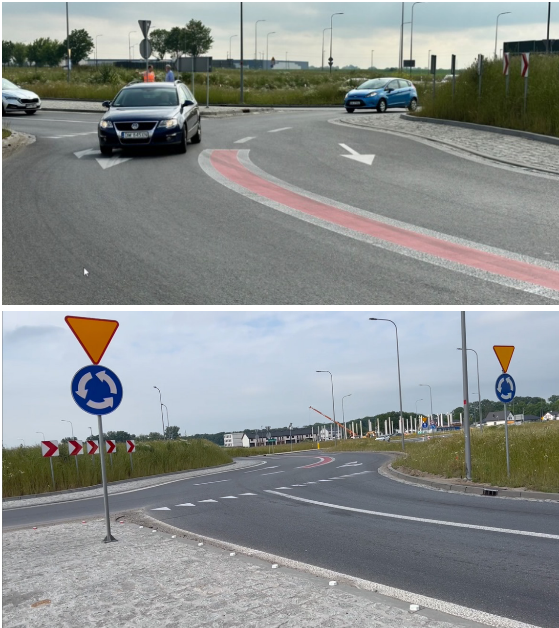
Figure 4: Examples of painted lane separation markings in the circulatory roadway in Poland (Source: FHWA)
