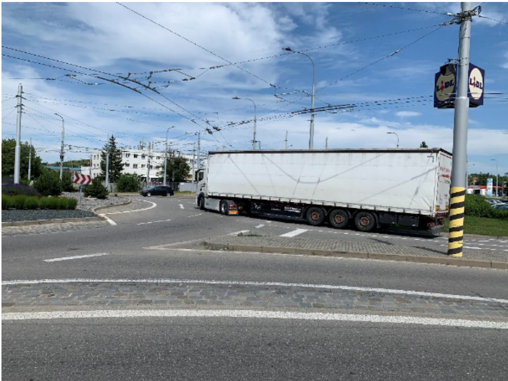
Figure 8: Raised channelization at the exit of a turbo roundabout in the Czech Republic (Source: FHWA)
