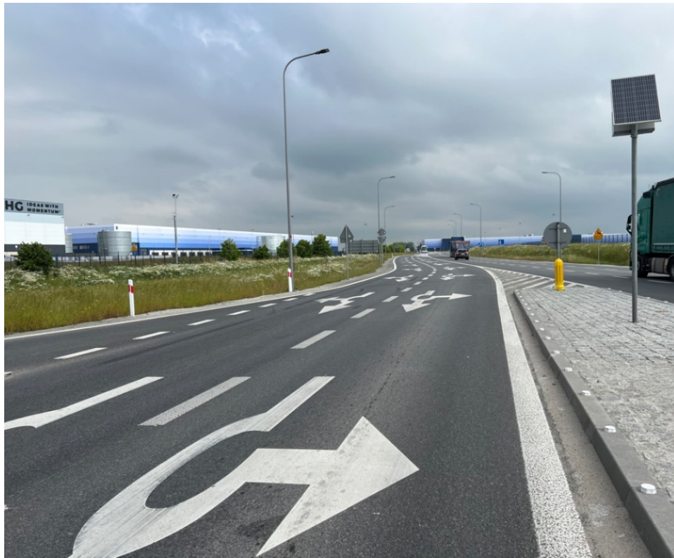
Figure 17: Series of approach pavement markings (distance based on expected queue length) in Poland (Source: FHWA)
