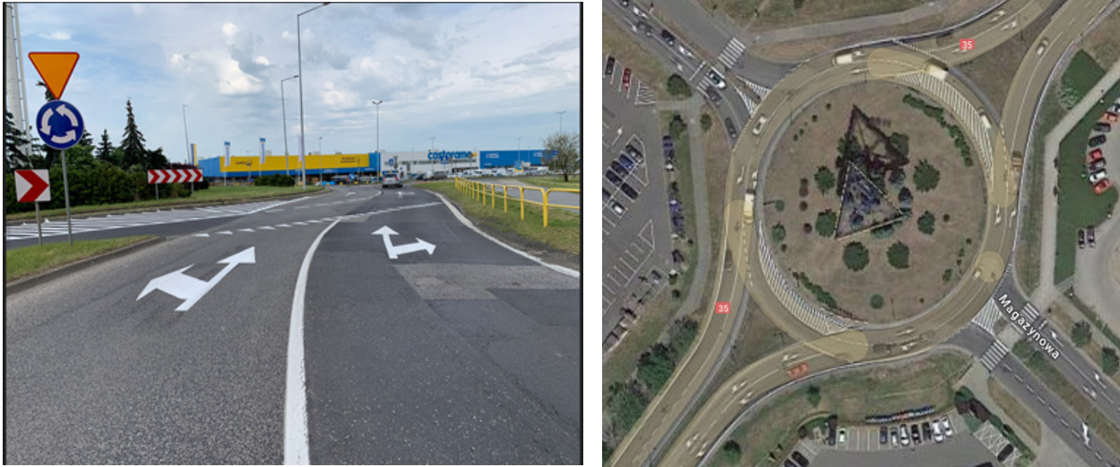
Figure 34: Ground level and aerial views of a retrofitted turbo roundabout near Wroclaw, Poland (Source: FHWA and Google Maps)
