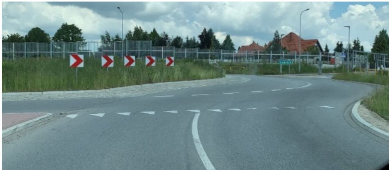
Figure 3: Example of approach lane markings in Poland (Source: FHWA)
