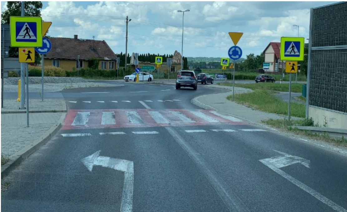
Figure 20: Rural turbo roundabout with a rounded inner lane center island in Poland (Source: FHWA)
