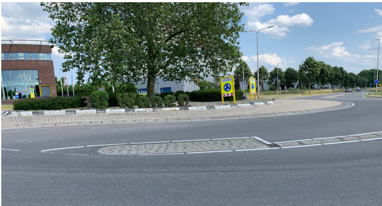
Figure 6: Raised channelization in the circulatory roadway at a rounded inner lane center island in the Netherlands (Source: FHWA)
