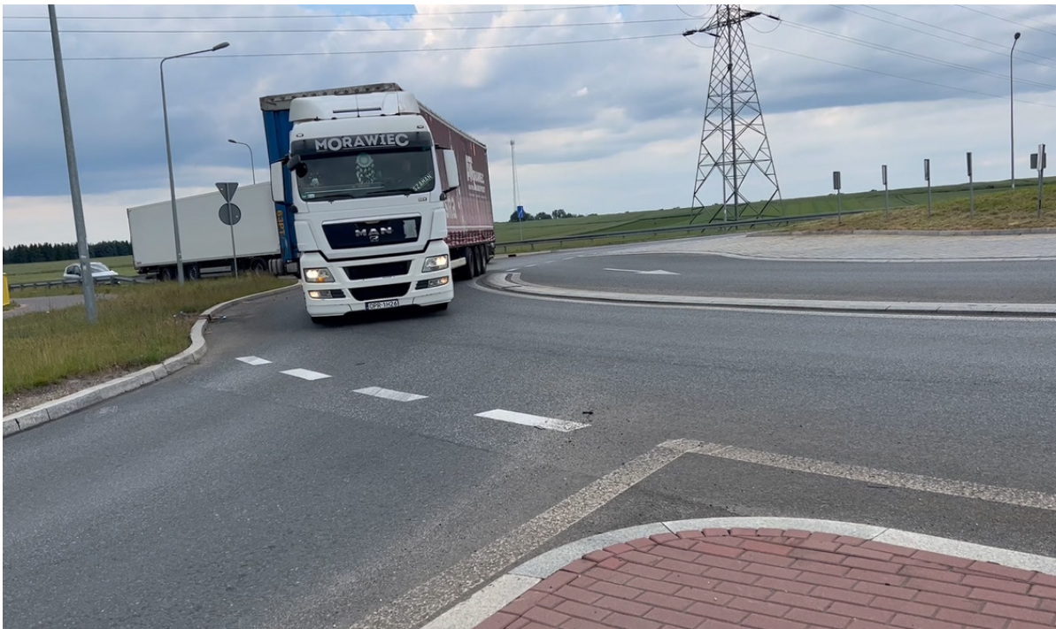
Figure 29: A truck traveling through a turbo roundabout interchange with raised channelization in the circulatory roadway in Poland
