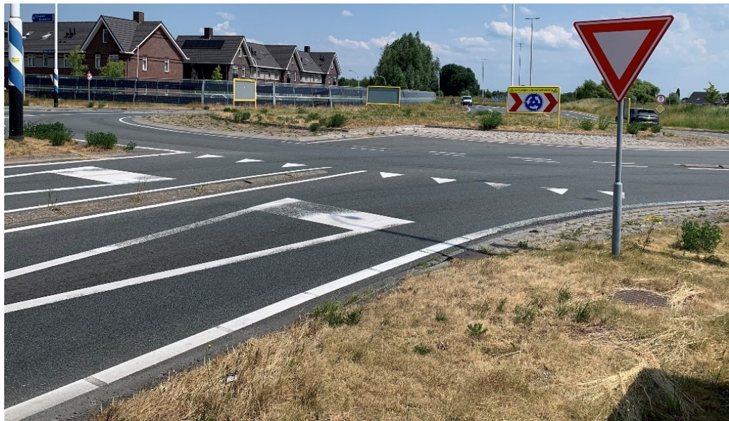
Figure 10: Example of basic pavement markings and a raised lane divider within the approach in the Netherlands (Source: FHWA)
