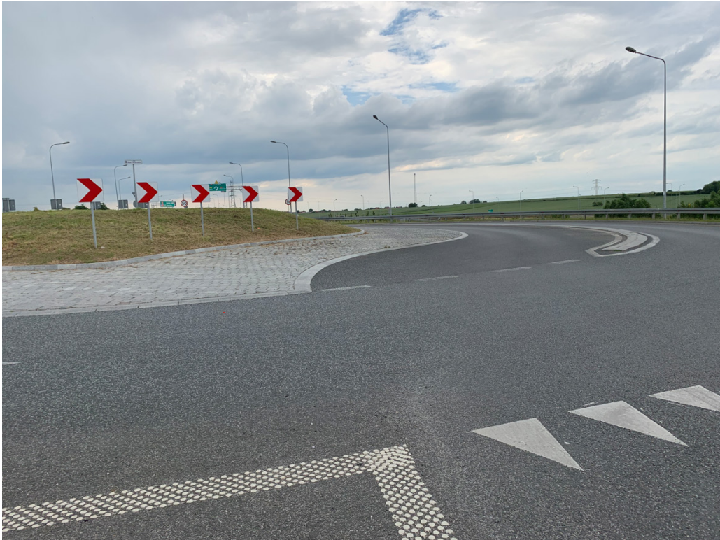
Figure 7: Raised channelization in the circulatory roadway at a rounded inner lane island in Poland (Source: FHWA)
