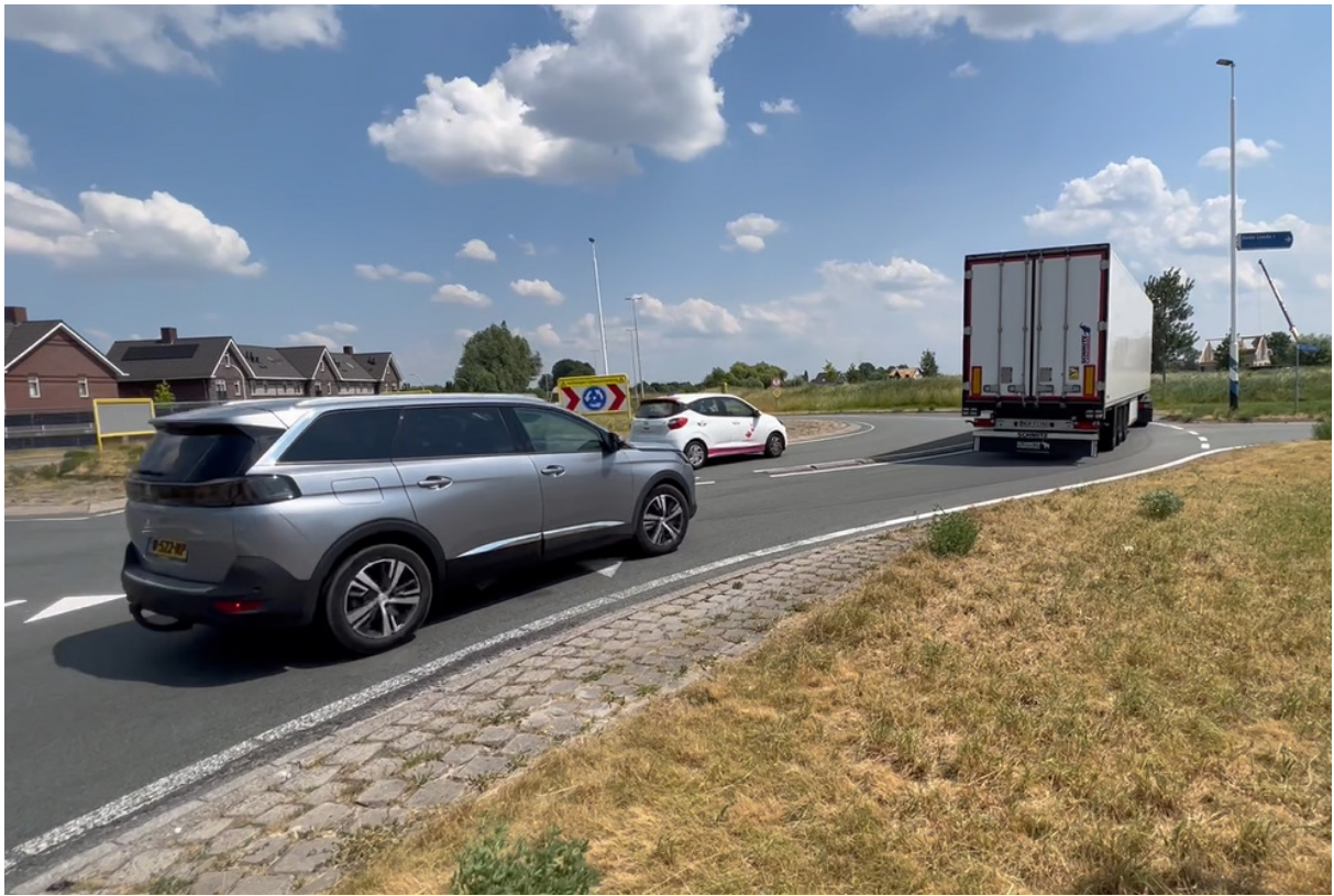
Figure 28: Vehicles traveling side-by-side with raised channelization in the Netherlands (Source: FHWA)
