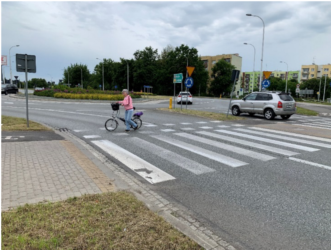
Figure 24: Separated pedestrian and bicycle pathway crossings in Poland (Source: FHWA)
