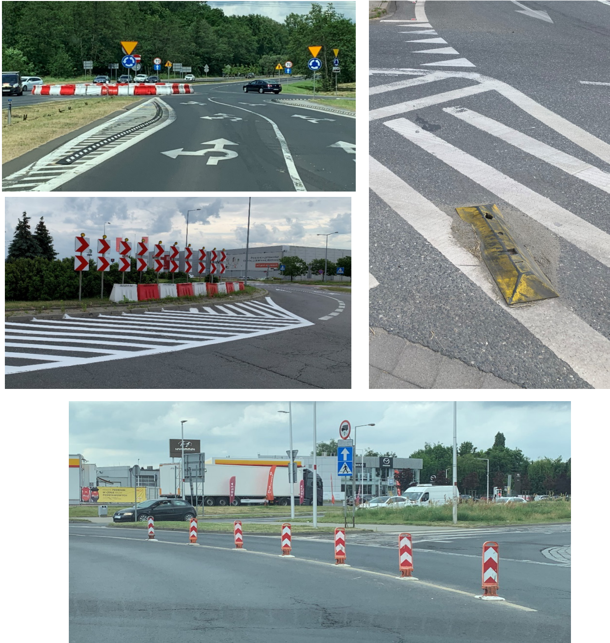
Figure 35: Examples of temporary lane delineators used to retrofit roundabouts in Poland (Source: FHWA)
