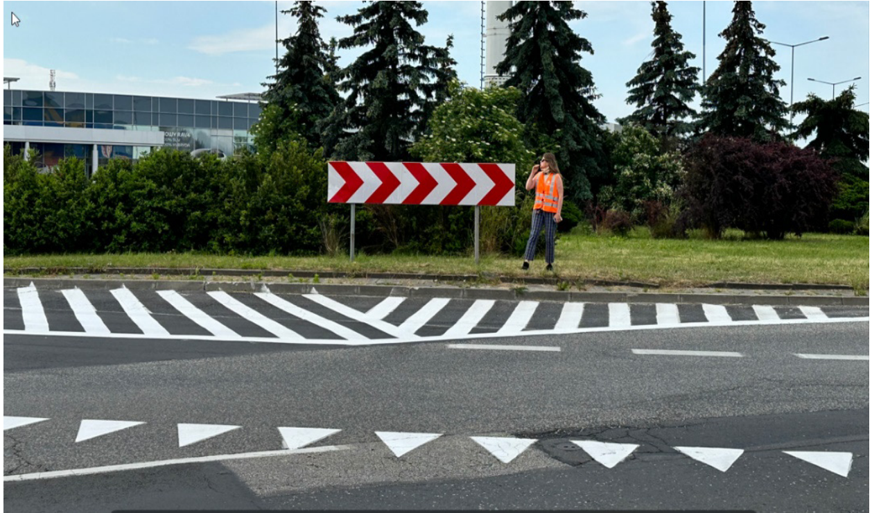
Figure 15: Large directional arrows in the center island of a retrofit turbo roundabout in a freight corridor in Poland (Source: FHWA)
