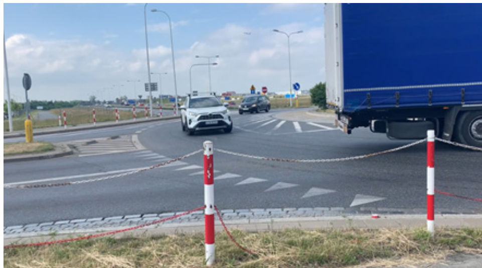
Figure 33: A retrofitted turbo roundabout near Wroclaw, Poland (Source: FHWA)
