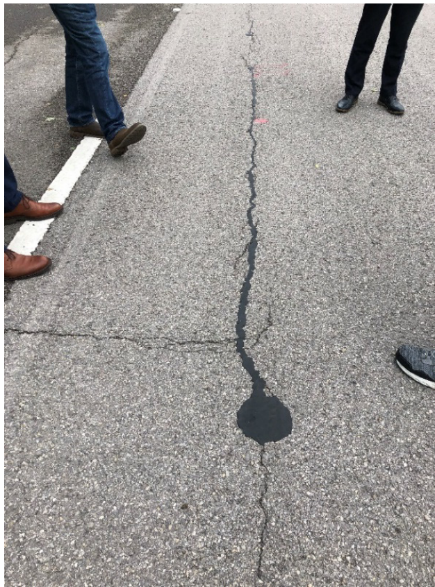
Figure 6. National Highways Smart Motorways Development Centre – UAS Enhancing Pavement Preservation
