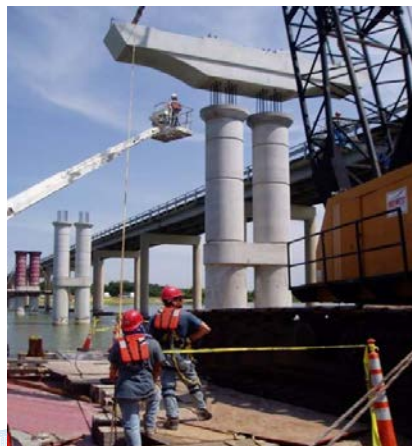
Figure 32. Installation of precast cap in the Lake Belton Bridge.
