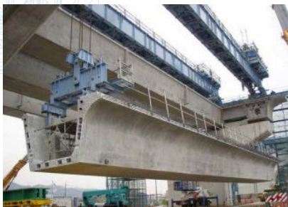
Figure 34. Erection of a precast U-girder.
