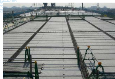
Figure 35. Installation of precast panels.
