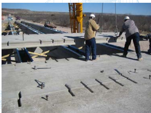
Figure 33. Erection of full-depth precast panels in the Live Oak Creek Bridge.
