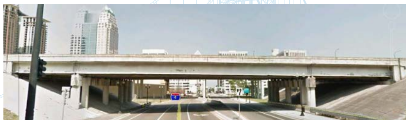
Figure 24. A bridge in Orlando assessed by IR technology.
