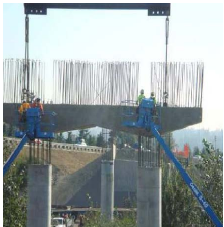
Figure 31. Installation of precast bent cap in Washington.
