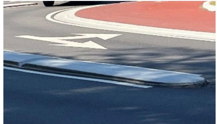
FIGURE 3. RAISED PAVEMENT CHARACTERISTICS OF TURBO ROUNDABOUT. SOURCE: FHWA
