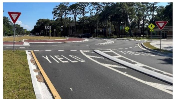
**FIGURE 2.** APPROACH CHARACTERISTICS OF TURBO ROUNDABOUT IN JACKSONVILLE, FLORIDA. **SOURCE:** FHWA
