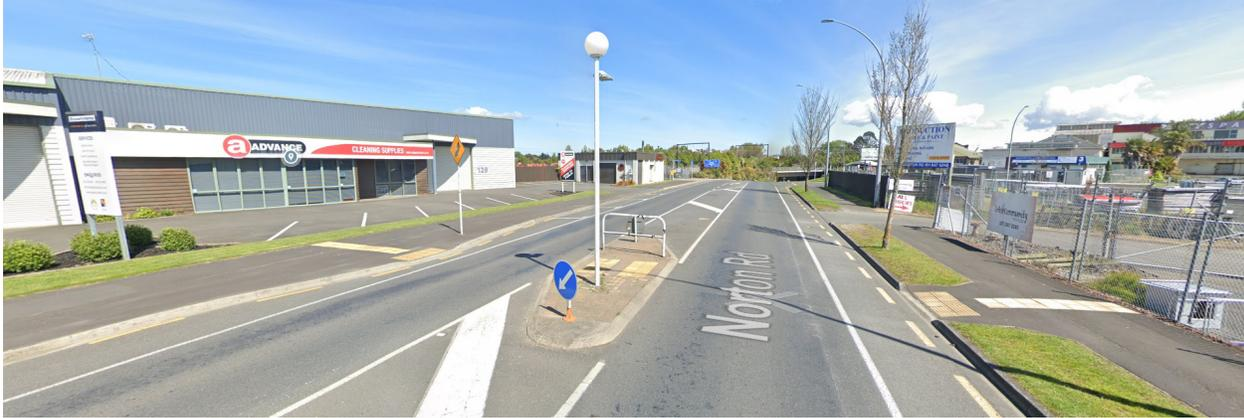
Figure 6: Norton Road with protected median refuge including a raised island, signs, overhead lighting, curb cuts, and tactile dome warning strips (Source: [Google Maps](#))
