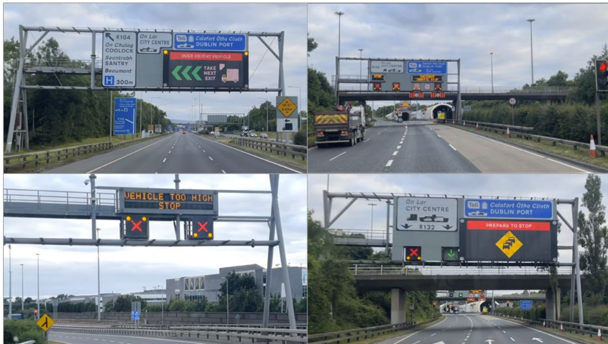
Figure 11: Transport Infrastructure Ireland Tunnel Over-Height Warnings and Closure
