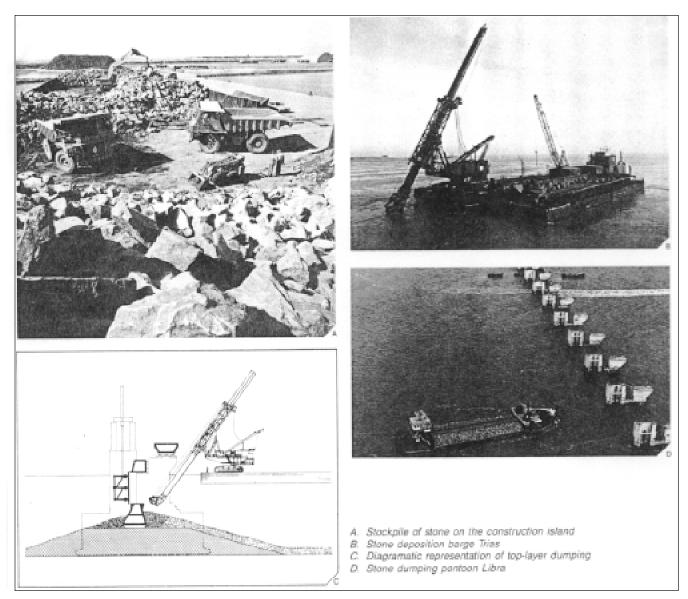
Figure 9. Armor stone and specialized stone placing equipment—Eastern Scheldt Barrier, the Netherlands (26).
