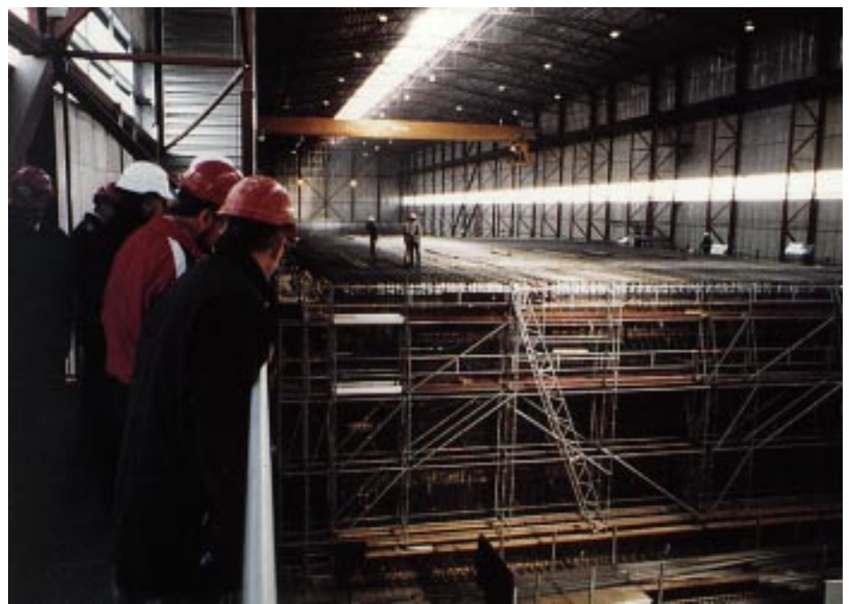
Figure 2. Inside the casting facility at the Øresund Link Project.
