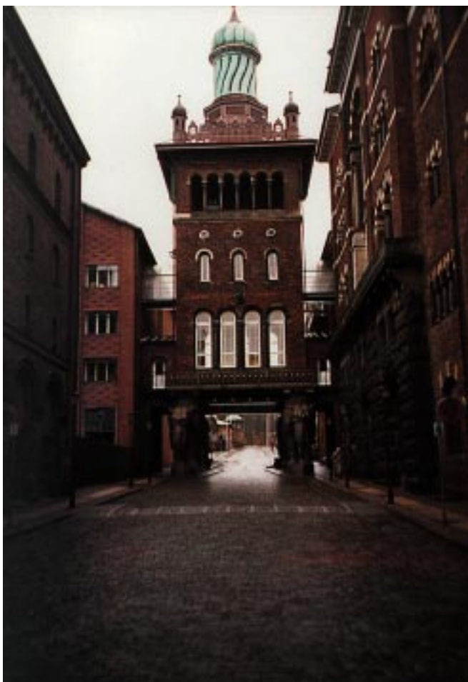
Figure 10. Interesting foundation approaches were also observed.
