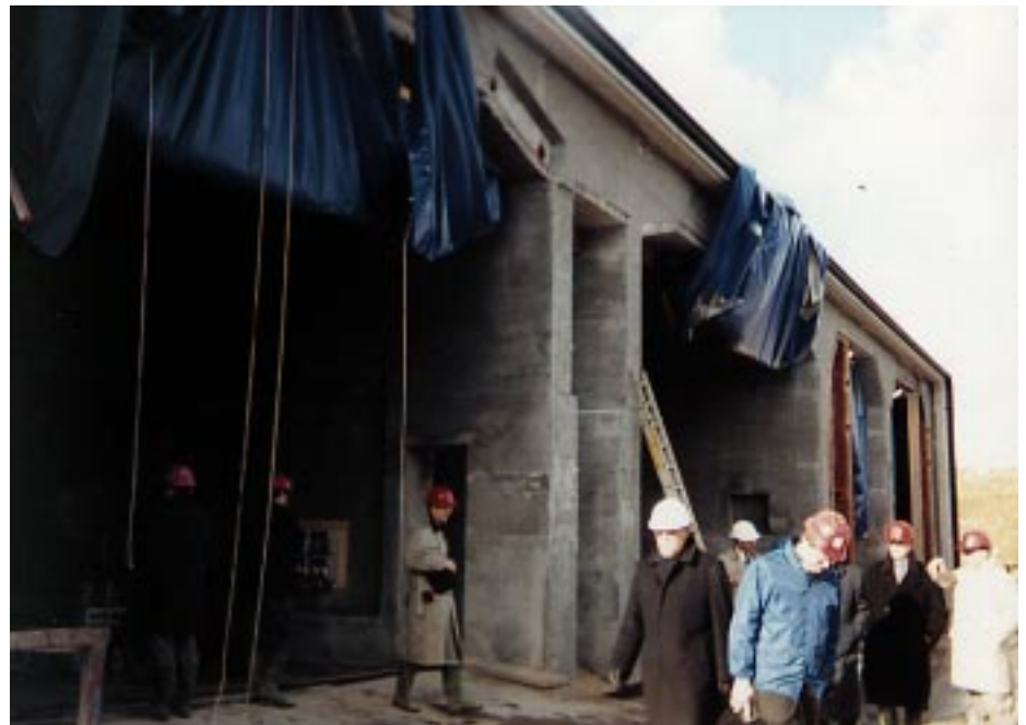
Figure 3. Tunnel element being pushed out of the casting area.
