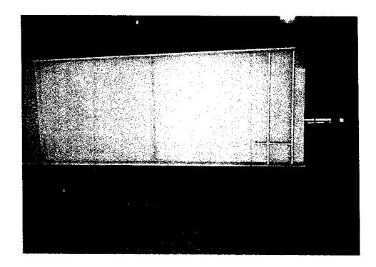
Figure 13. Finished metalized girder before sealing with topcoats.
