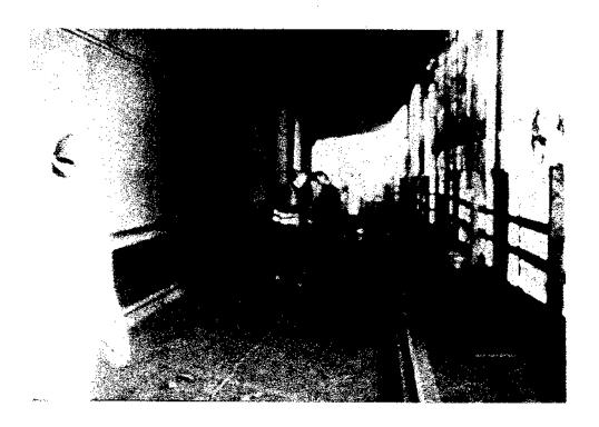
Figure 3. View inside large containment structure, Haseltallbrucke, Germany. Note rails for mobile scaffolding, rigid flooring, and facia girder on left.
