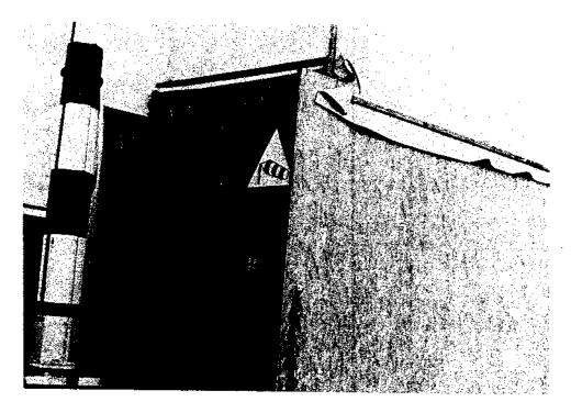
Figure 5. Rigid entry doorway to containment structure in the Netherlands. Note the foam sealing the seams and the "lead" pencil warning sign above the fixed hinged doorway.
