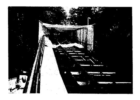
Figure 2. View of containment on steel tram structure, Zurich, Switzerland
