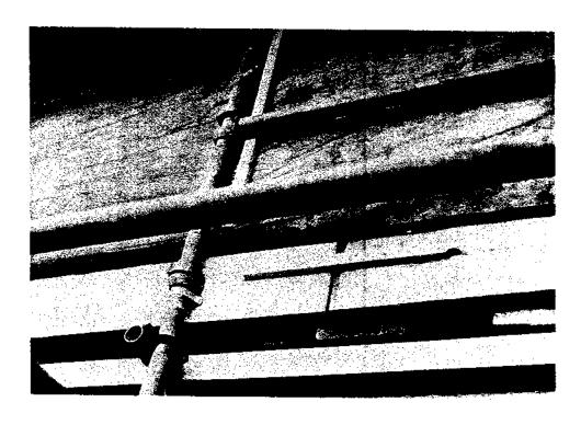
Figure 4. Mechanically fastened joints in containment tarps. All joints are nailed closed with wooden supports.
