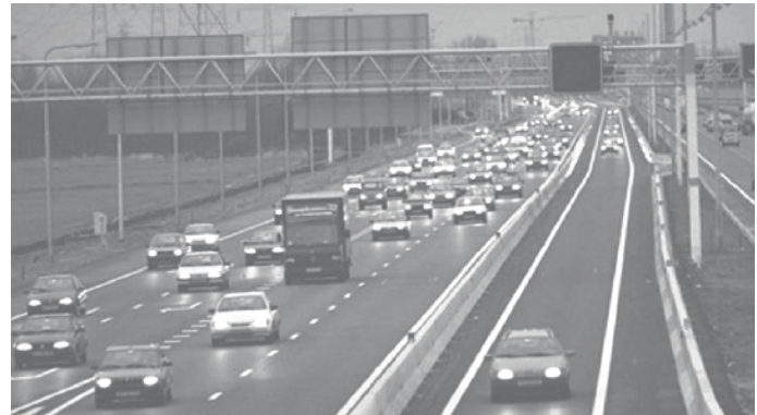
Figure 42. Tidal flow lane in the Netherlands. (45)
