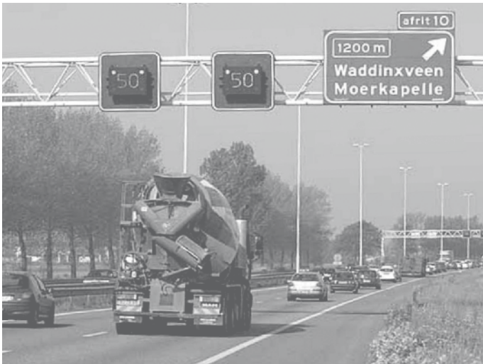
Figure 33. Congestion warning system in the Netherlands. (45)
