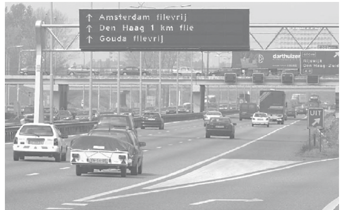
Figure 41. Dynamic route information panels in the Netherlands. (45)
