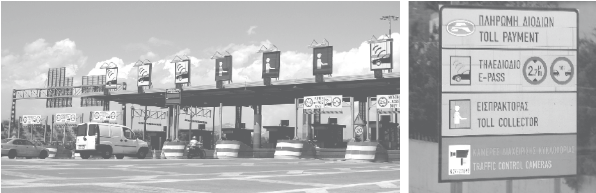
Figure 7. Attiki Odos toll plaza (left) and related plaza sign (right) in Athens, Greece.
