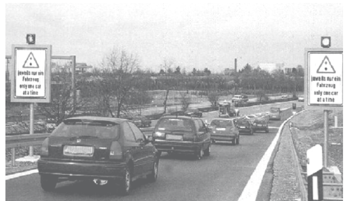
Figure 21. Ramp metering in Germany. (26)
