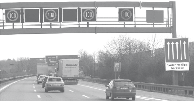
Figure 15. Right shoulder use with speed harmonization in Germany. (29)
