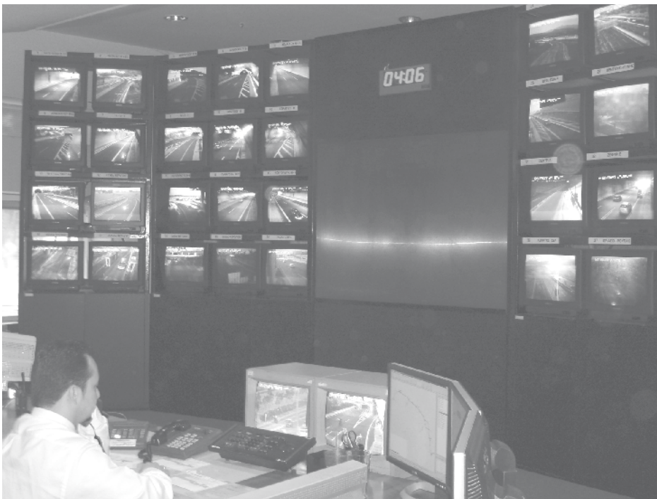
Figure 8. Attiki Odos Traffic Management Center in Athens,
