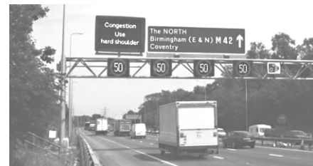
Figure 49. M42 ATM with hard shoulder running. (58)
