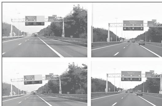
Figure 35. Temporary right shoulder use in the Netherlands. (49)
