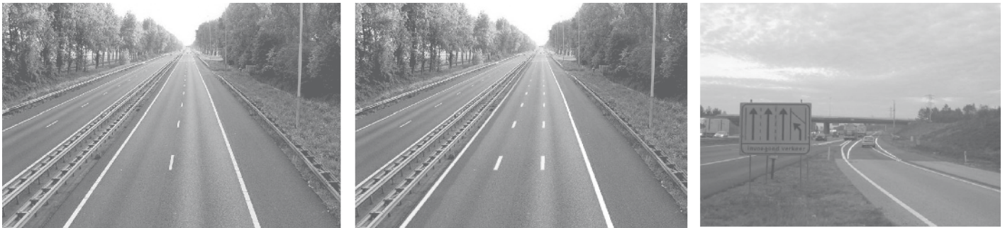
Figure 38. Dynamic lane marking in the Netherlands. (45,49)
