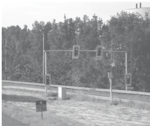
Figure 40. Ramp metering in the Netherlands.
