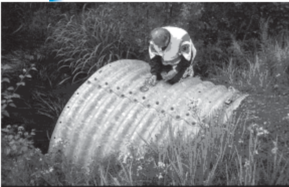
Figure 8. Ultrasonic thickness inspection in Finland.
