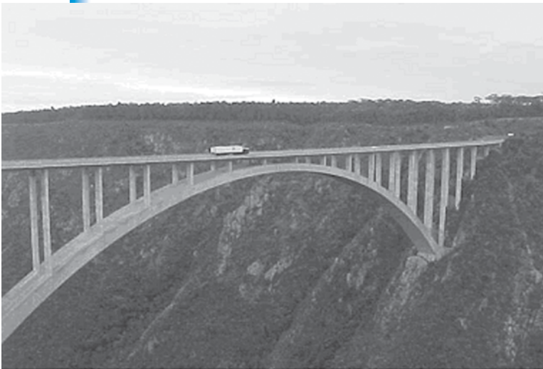
Figure 29. South African highway bridge.
