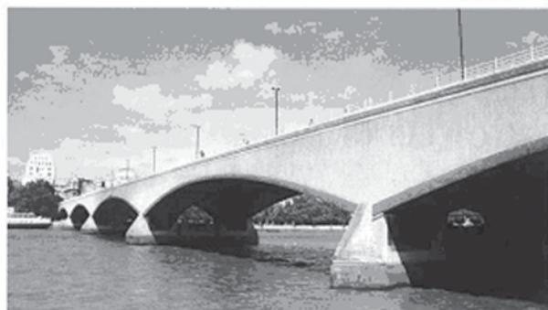
Figure 50. Waterloo Bridge. (Highways Agency 2003)
