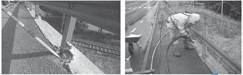
Figure 45. Measurement and maintenance of bridge railing.
