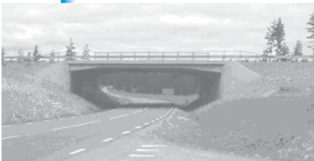
Figure 38. Swedish bridge with no joints or bearings.
