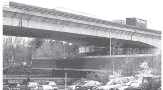
Figure 54. Railway viaduct at Huntingdon.
