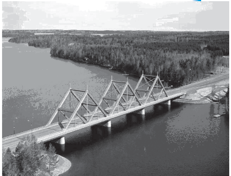
Figure 9. Finland's Vihantasalmi Bridge.
