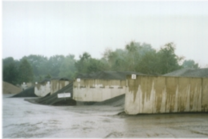
Figure 13. RAP bins for use at DEUTAG hot mix asphalt plant in Germany.
