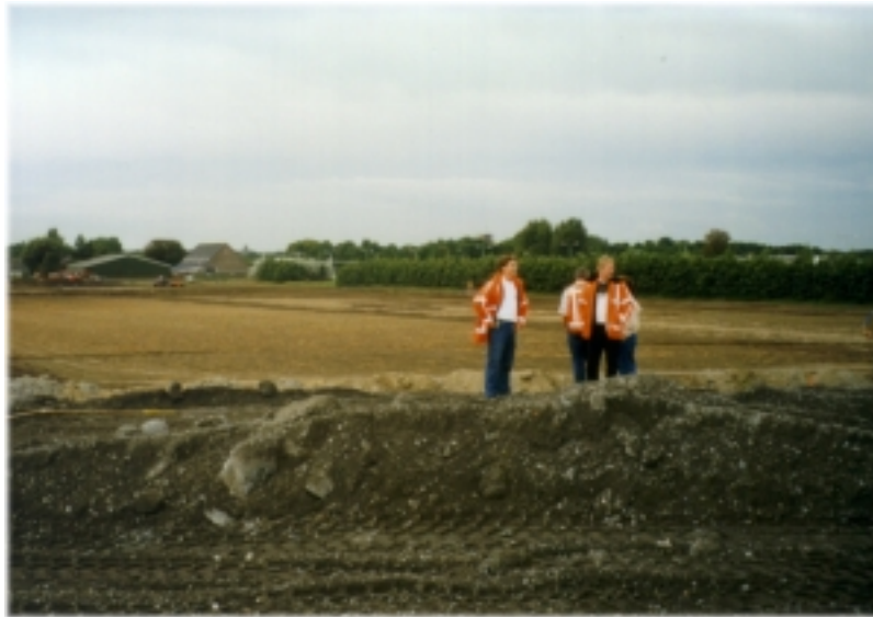
Figure 19. WTE bottom ash use in a road embankment in the Netherlands.
