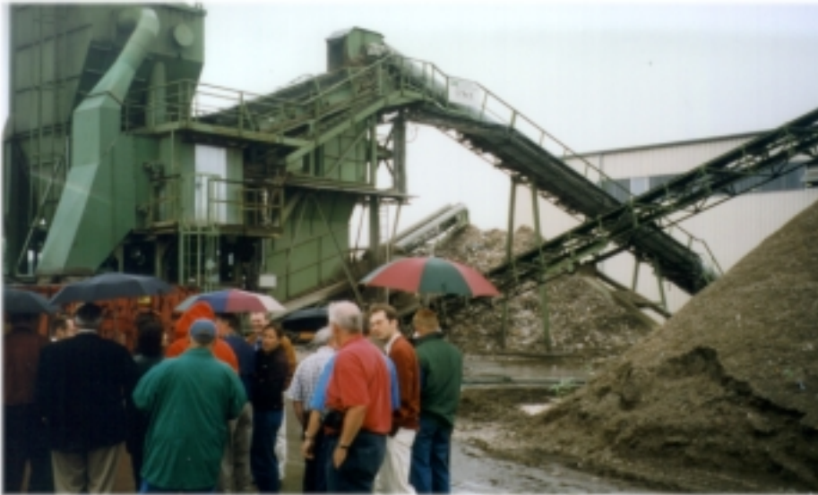
Figure 17. Aggregate crushing and sorting facilities at the Remex C&D processing plant. The pile in the foreground is aggregate made from crushed C&D waste. It will be used in highway base course.
