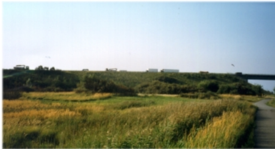
Figure 9. A highway bridge embankment constructed with coal fly ash in Denmark.
