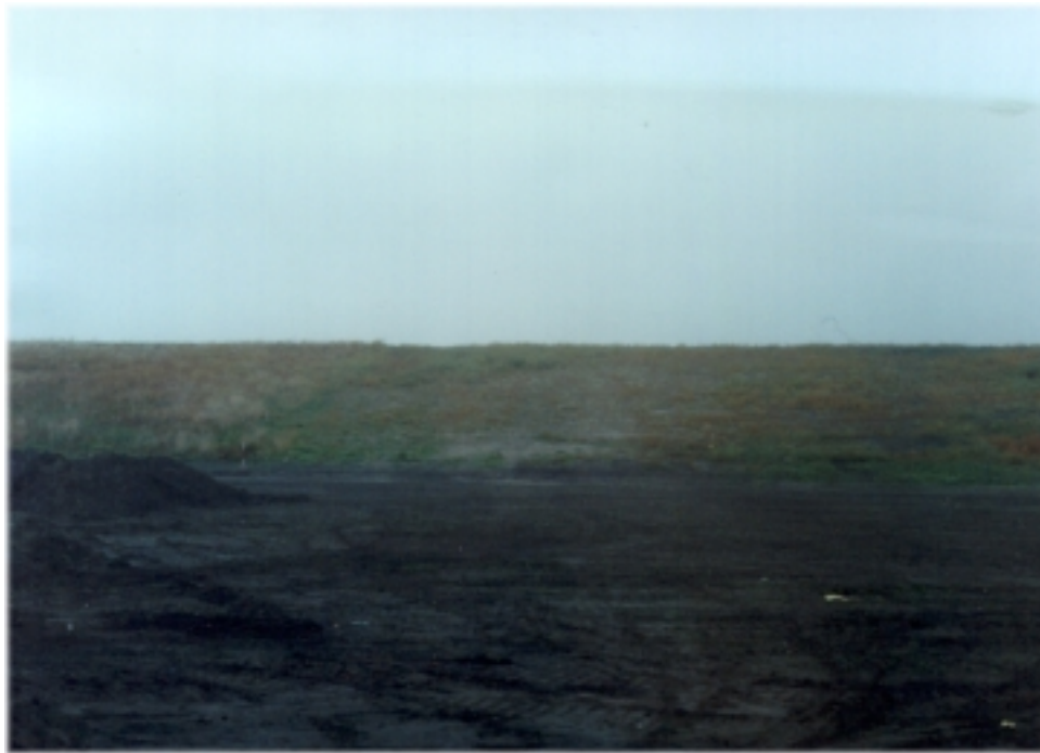
Figure 18. The noise control embankment at Ypenburg in the Netherlands. The barrier is made with lightly contaminated soils.
