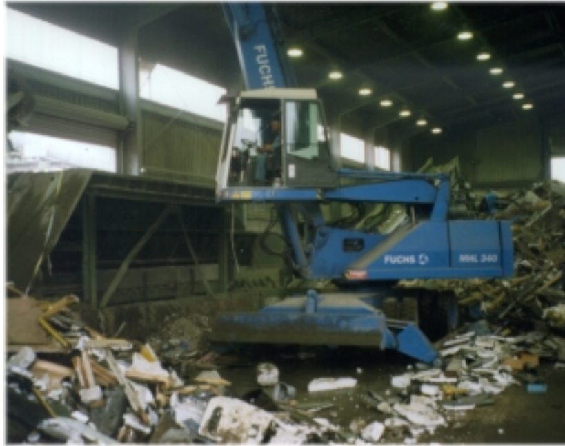
Figure 15. C&D wastes to be processed at the Remex C&D processing plant in Germany.
