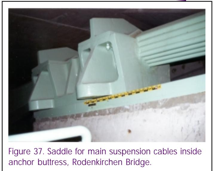
Figure 37. Saddle for main suspension cables inside anchor buttress, Rodenkirchen Bridge.
