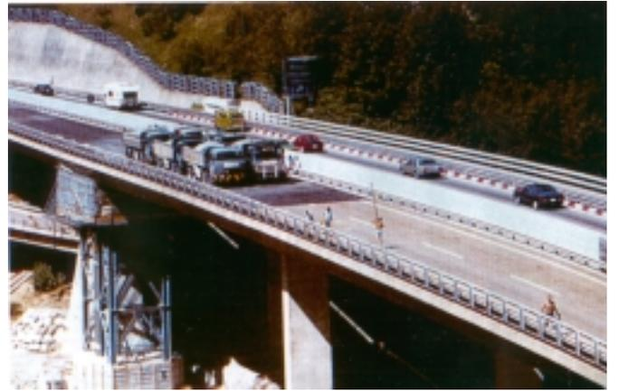
Figure 22. The pier of Reuss Bridge was shored-up, the post-tensioned box superstructure was jacked up to level, repaired, and load-tested.
