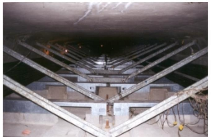
Figure 29. Internal frames on Corbeil Bridge brace the bottom slab and webs. External longitudinal tendons run inside the box near the webs.
