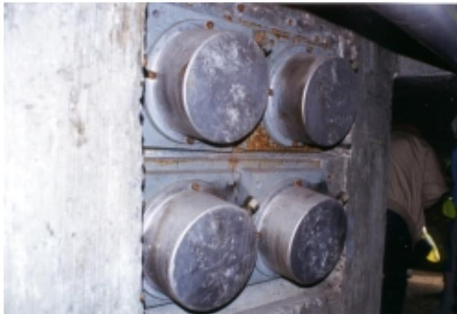
Figure 31. Anchor protection for new external tendons on Corbeil Bridge.
