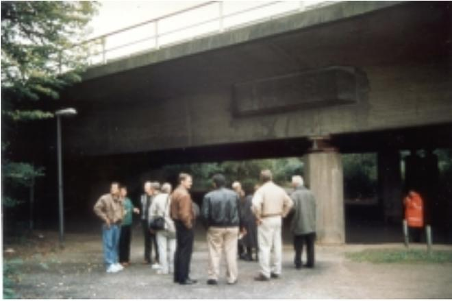
Figure 26. Scan team examines anchor blocks for external tendon retrofit of L124 viaduct.
