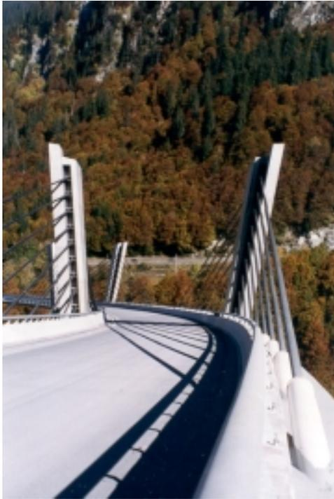
Figure 6. On the Sunniberg Bridge, short pylons rise away from the deck to accommodate the curve of the highway.
