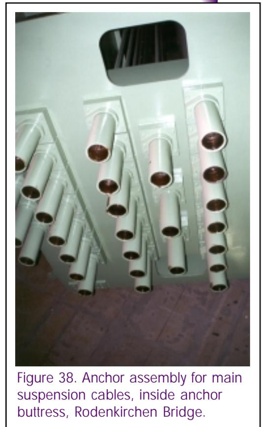
Figure 38. Anchor assembly for main suspension cables, inside anchor buttress, Rodenkirchen Bridge.
