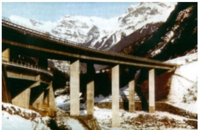
Figure 23. The reconstructed Reuss Bridge was re-opened in 1988. This case demonstrates the advantages of the inherent redundancy of continuous, post-tensioned, concrete construction.
