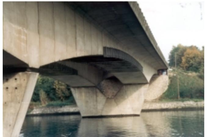
Figure 28. The Corbeil Bridge, Francillienne, Essone, France, on which external transverse post-tensioning was added to the midspan region.
